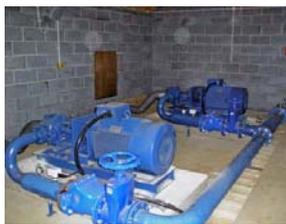
system varies the speed of the pump to meet water demand and pressure, using less energy when fewer irrigation reels are running. This system comes with a touch screen control as
